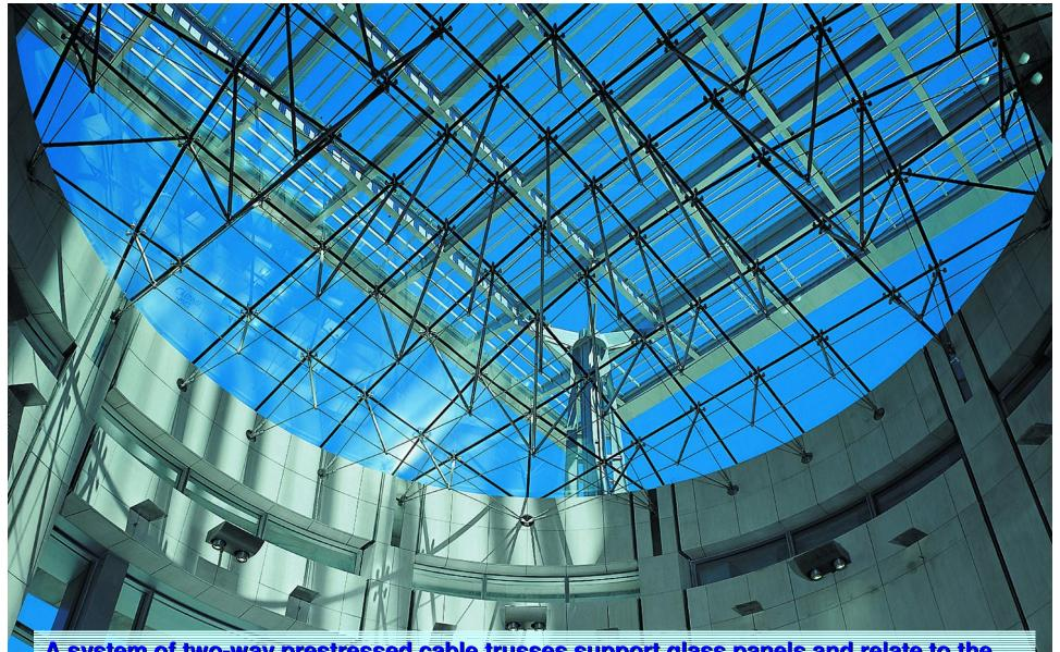
A system of two-way prestressed cable trusses support glass panels and relate to the irregular surface geometry.
