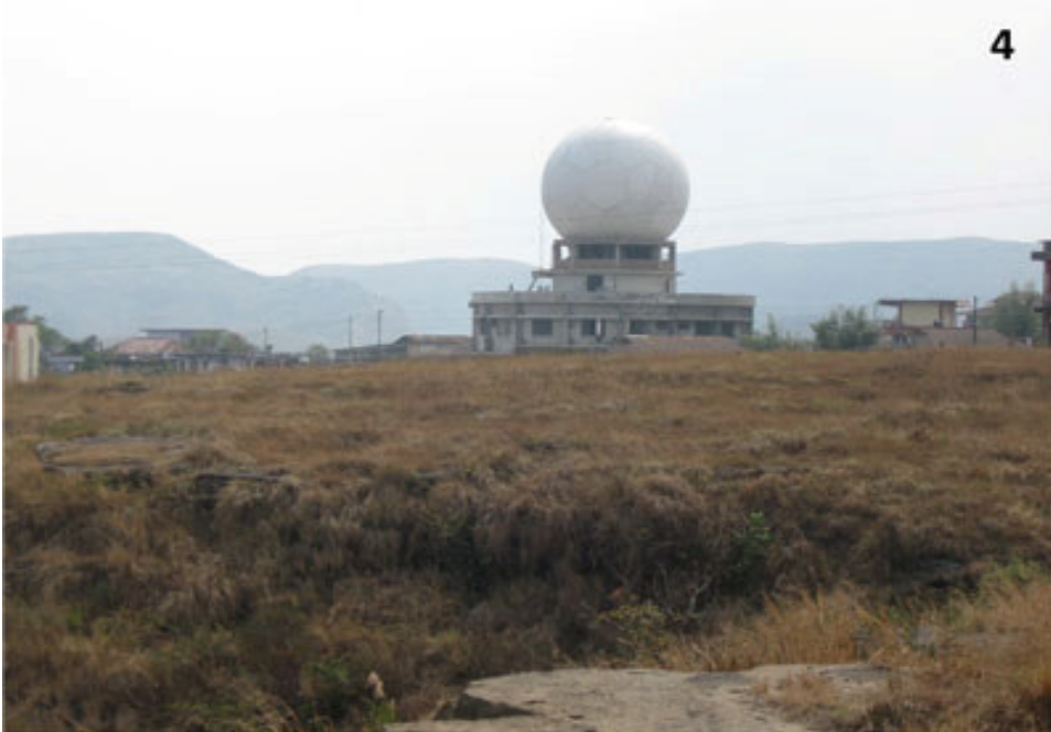
Figure 4. View of the fully assembled Radome from a distance
