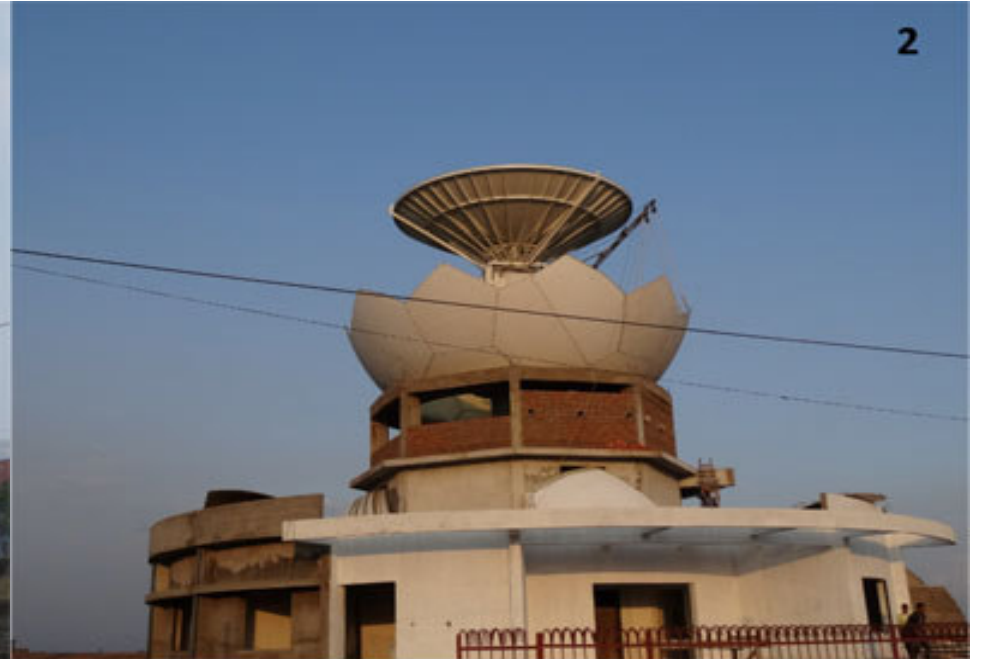
Figure 2. CSIR-NAL's DWR Radome assembly below the equator level
